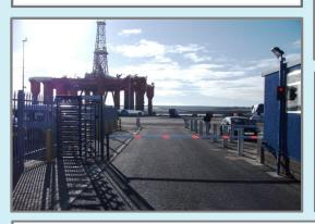
The final installation consisted of automated gates and barriers, pedestrian turnstiles, voice, video and keypad intercoms, automated license plate recognition, and an extensive high definition CCTV system complete with both static and PTZ cameras – several of which broadcast via a wireless network due to geographical constraints on site.
